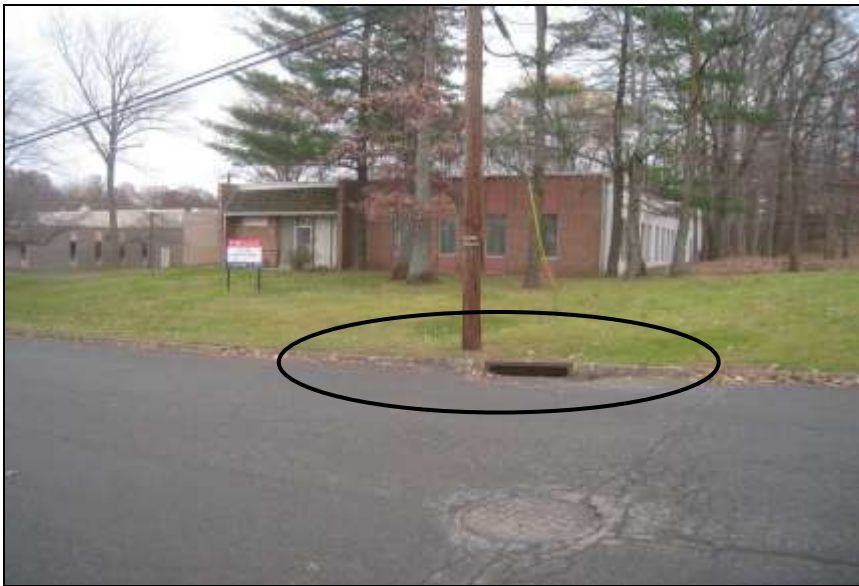
Photo # 7- Observed storm drain just past SW corner of building along Russo Place.
